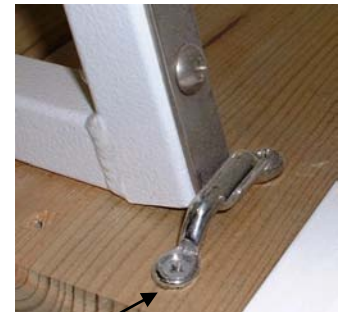
FOOTMAN'S LOOP ATTACHES TO DOCK
